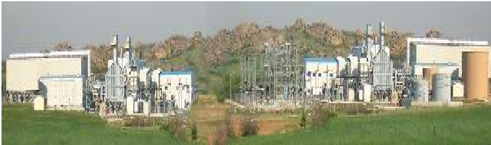
Kirklareli I and II Gas Fired Combined Cycle Power Plants, Kirklareli - Turkey
