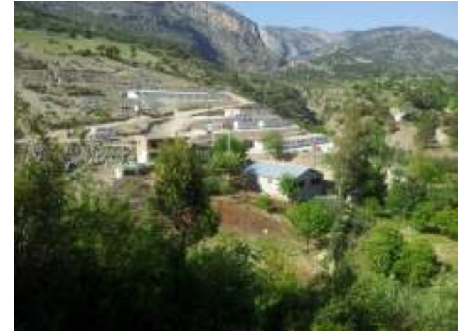
Karakuz Hydroelectric Power Plant Site View, Adana - Turkey
