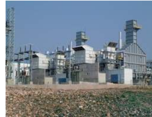
Kırklareli Power Plant, Kırklareli-Turkey
