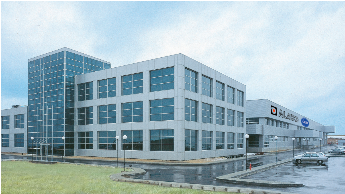
The Main Manufacturing Plant - Gebze
